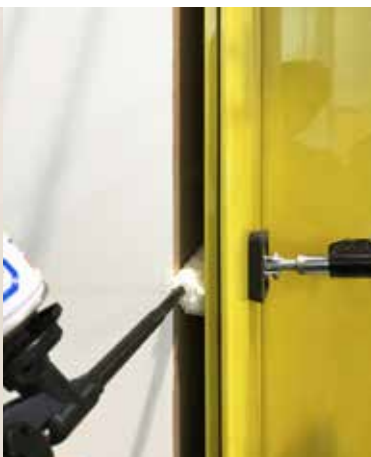
Anchoring with mounting foam
