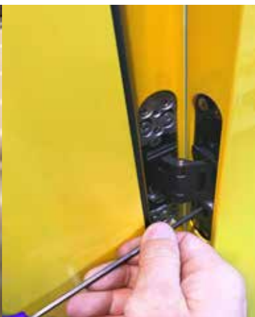
Installation of the hinges
