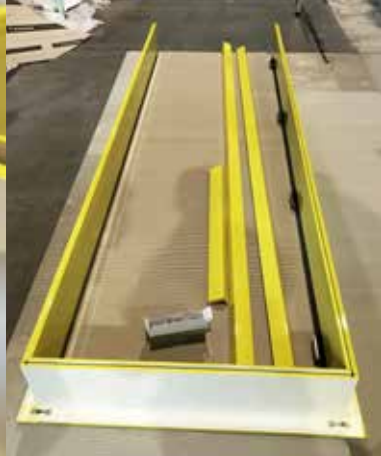
Completing the door frame
