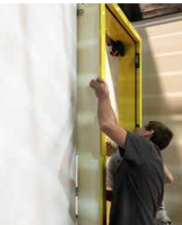
Fitting the door frame
