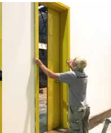
Installation of the target architrave
