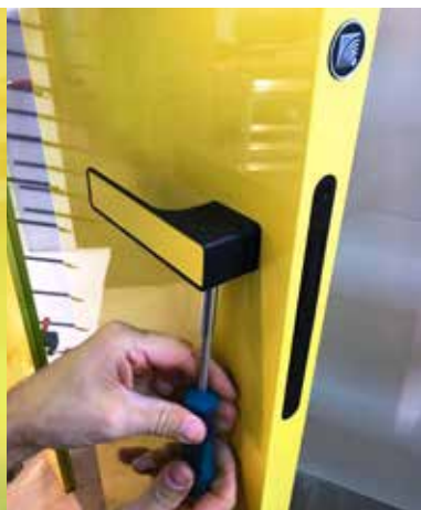
Installation of the handle
