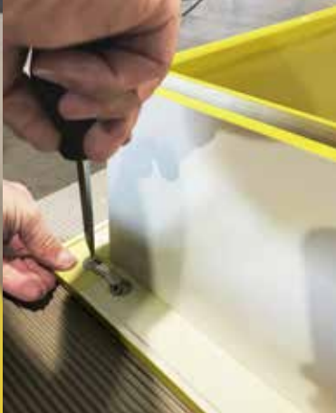
Fitting the door frame
